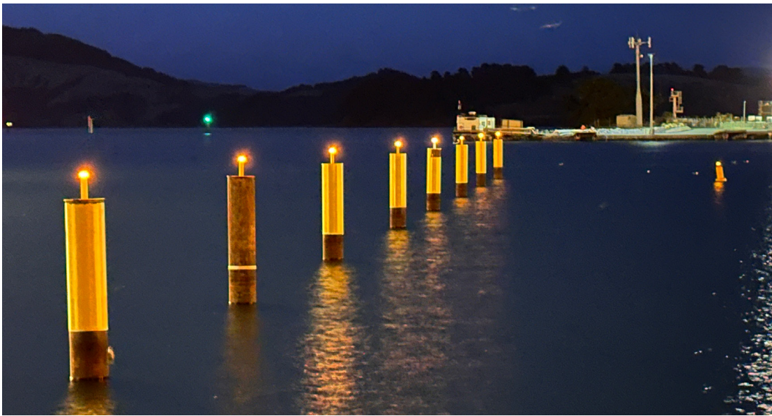
◀ Recently installed lights on steel piles indicate the shallow-water zone created by removing Jetties 4 and 5.
